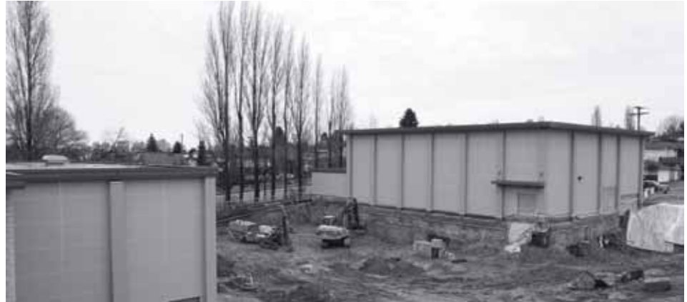
Recent Construction at ND
