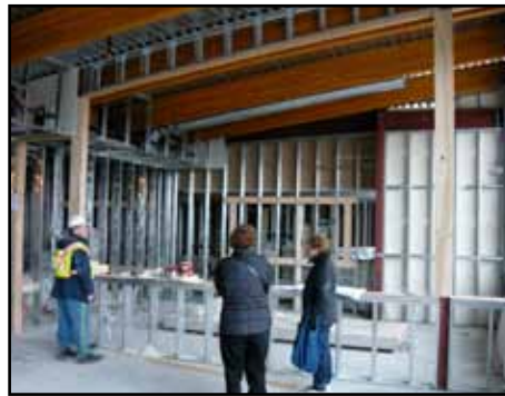
New school library meeting room underway
